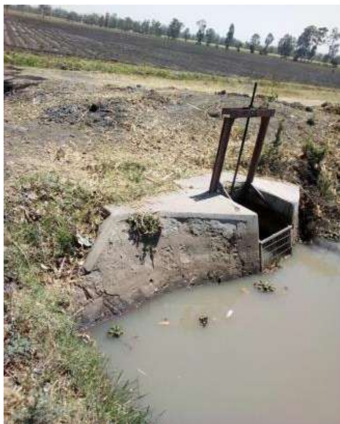
Plate 4: Outlet canal with mesh wire in Wonji reservoir, preventing escape of adult fish only.
